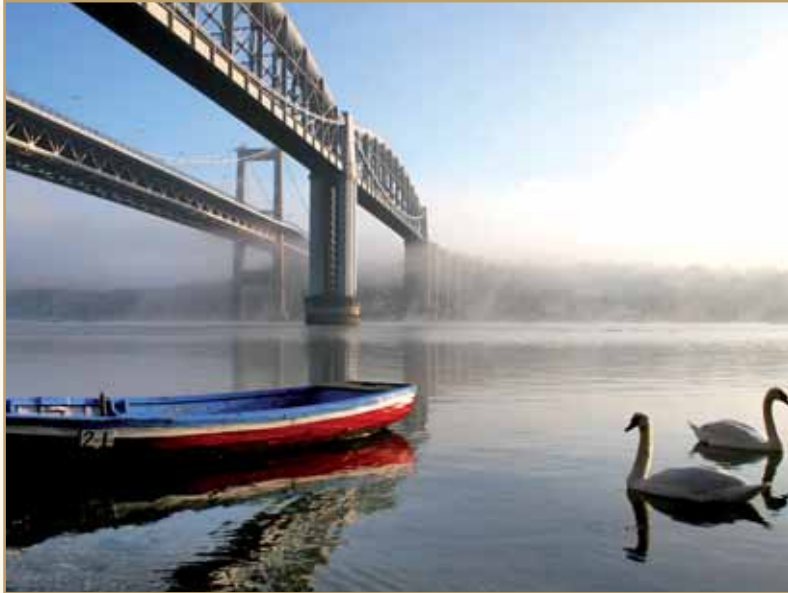
Bridges over the River Tamar
